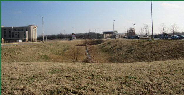
Site-specific storm water detention areas associated with the Hampton Inn and Lowe's commercial properties.
