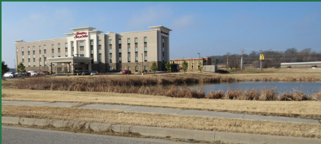
Site-specific storm water detention areas associated with the Hampton Inn and Lowe's commercial properties.
